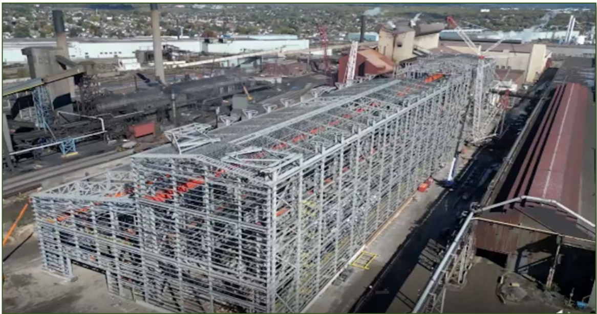
Photo 3: EAF 2 under construction, 2023-2024
